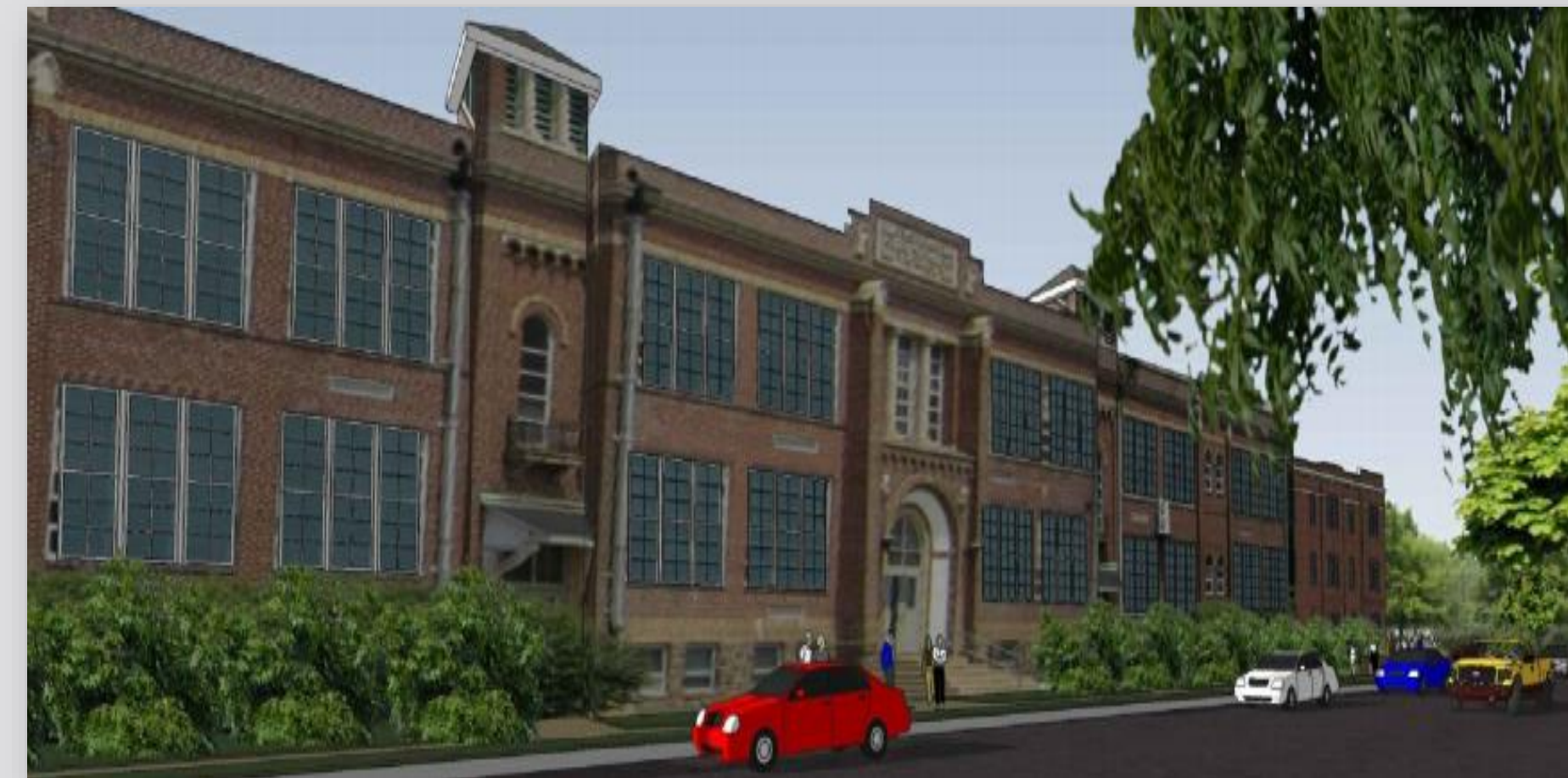
Provided by Gary Gardner Construction
